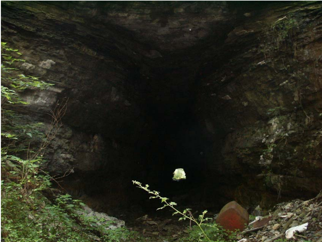
Photo 11. Abandoned Railroad Tunnel near Greensburg
