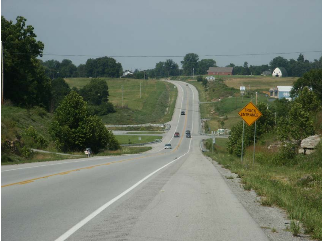
Photo 8. US 68 between Greensburg and Campbellsville in Green County
