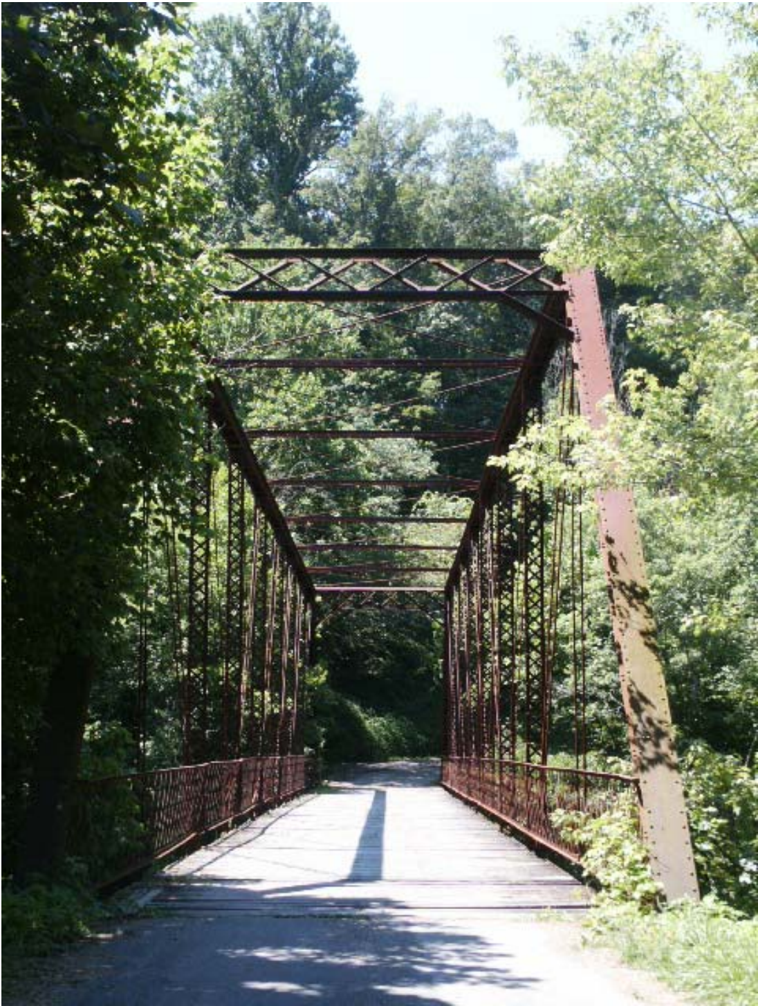
Photo 13. Historic Iron Truss Bridge over Green River
