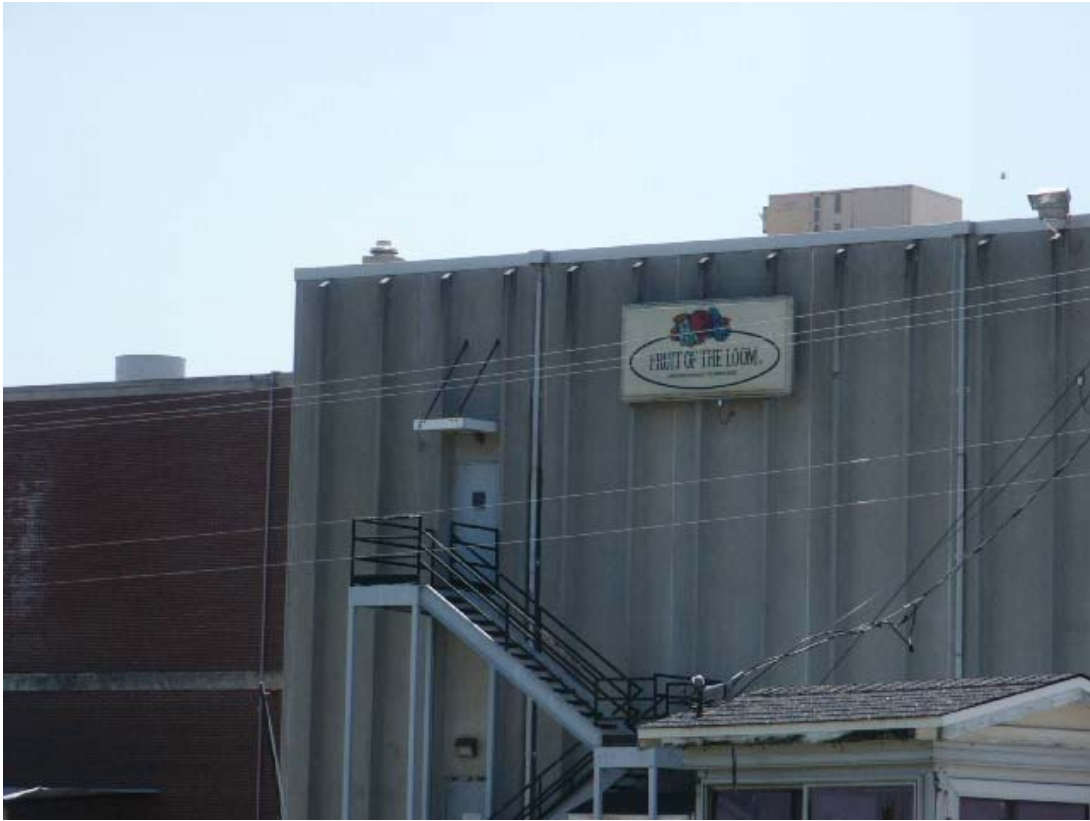
Photo 18. Former Fruit of the Loom plant in Campbellsville
